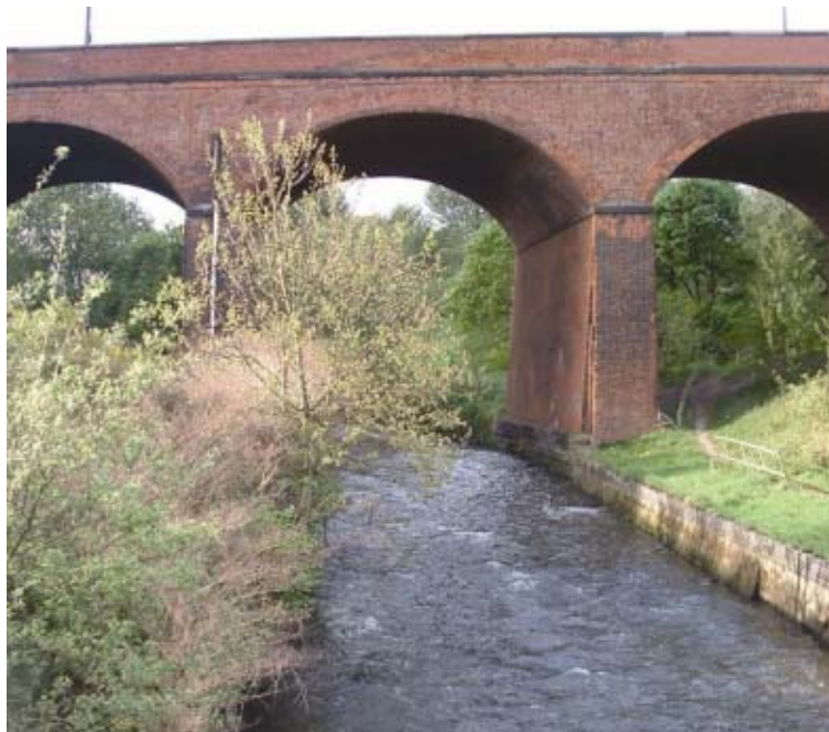
Figure 10 Viaduct over the Irk
